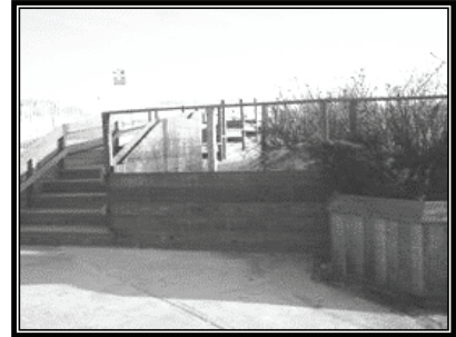
Newly renovated beach entrance at Pennsylvania Avenue
